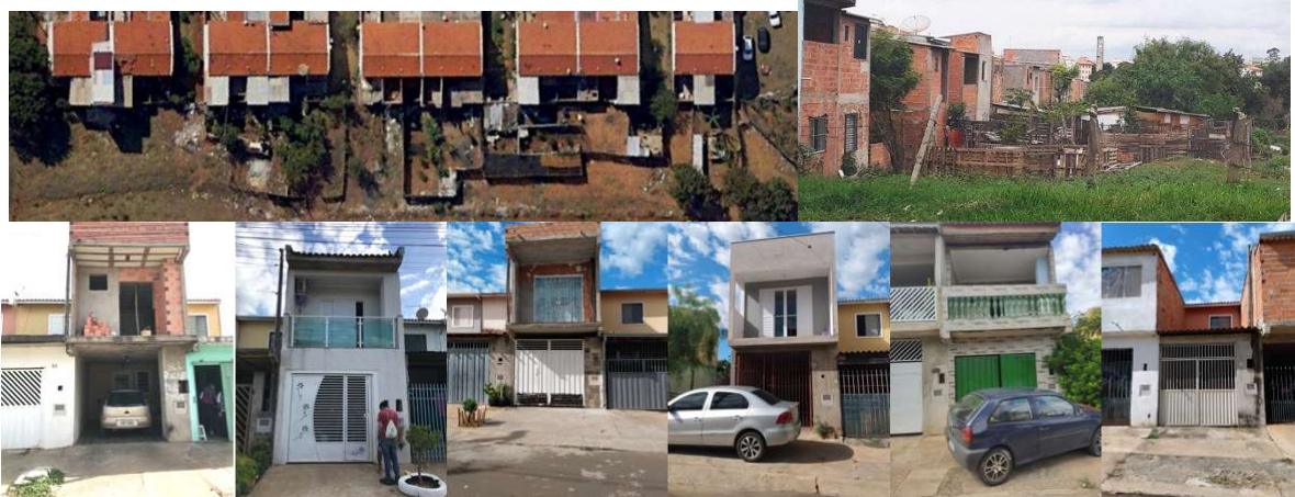
Figure 3: Transformations in Quilombo in 2022 (post-occupancy). Source: The authors
