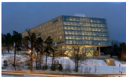
Figure 4: Think Tank – building view
