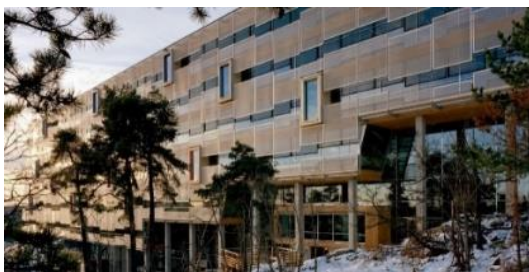
Figure 5: Think Tank – lateral façade view
